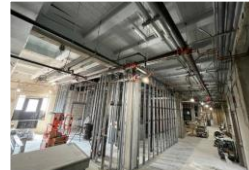
Mechanical Engineering Building Renovations
