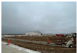
Airport Terminal Building
