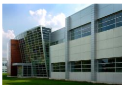
Birck Nanotechnology Center Clean Room Modernization and New Equipment
