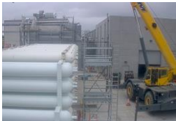
Zucrow High Speed Propulsion Lab
