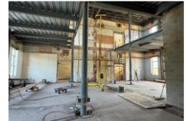
University Hall and Related Renovations
